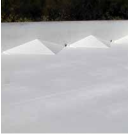
The ESP system conforms readily to the different shapes on a roof, as seen on the 'roof crickets' shown here.
