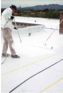
The ESP system conforms readily to the different shapes on a roof, as seen on the 'roof crickets' shown here.
