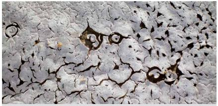
Example of damage caused by water intrusion on a foam roof.
